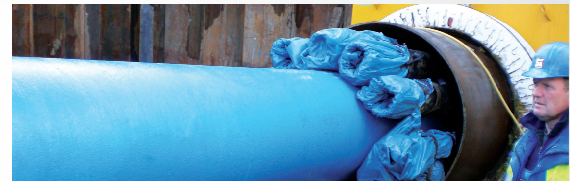
Ploughing-in a pipeline
