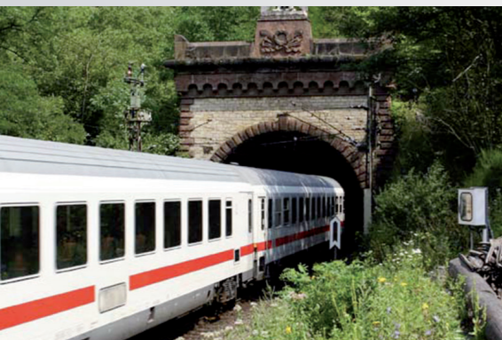
The Cochem Tunnel
