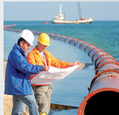
Floating in a ductile cast iron pipeline
