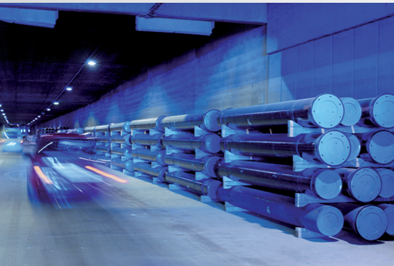
The Plabutsch Tunnel near Graz
