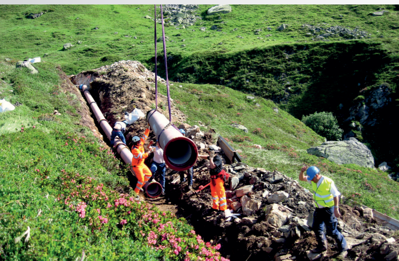
Laying in Alpine terrain
