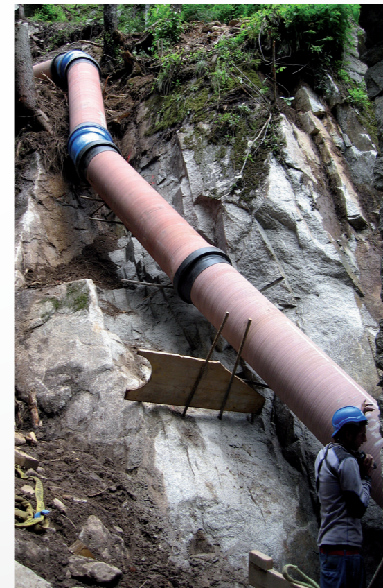
Laying on steep slopes
