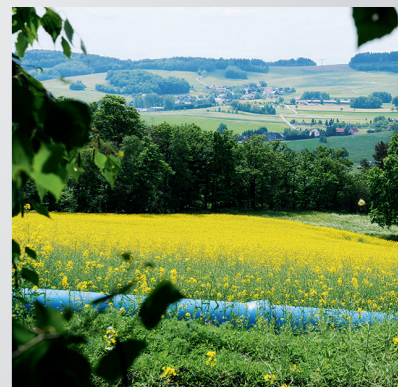
Temporary pipeline with VRS®-T/BLS® joints
