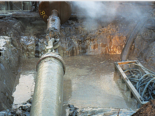
The horizontal directional drilling technique
