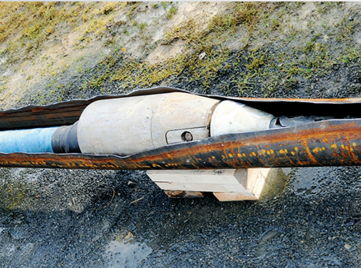
Above-ground demonstration of the burstlining technique
