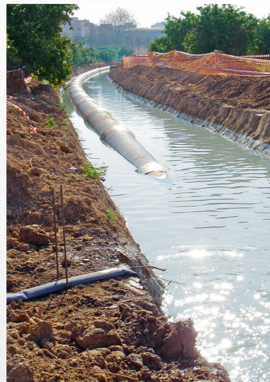
DN 900 directionally drilled curved pipeline in Valencia in Spain
