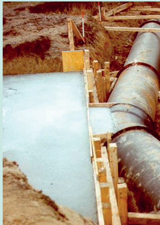
Conventional installation with concrete thrust block
